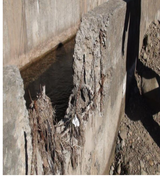
Seepage & Damages water Channel at various Points
