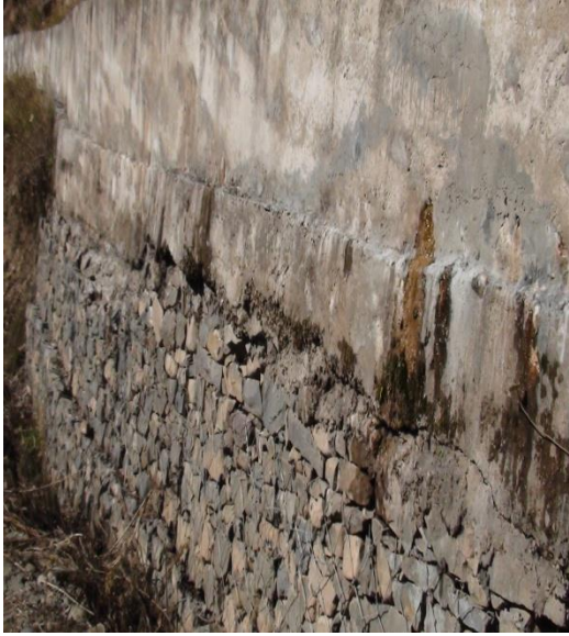
Seepage & Damages water Channel at various Points
