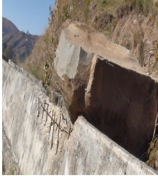
Water Channel Damage Due to Sliding
