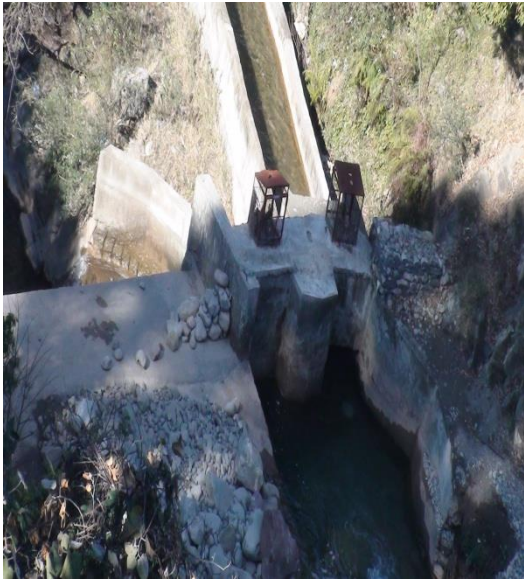
Inlet Water Channel
