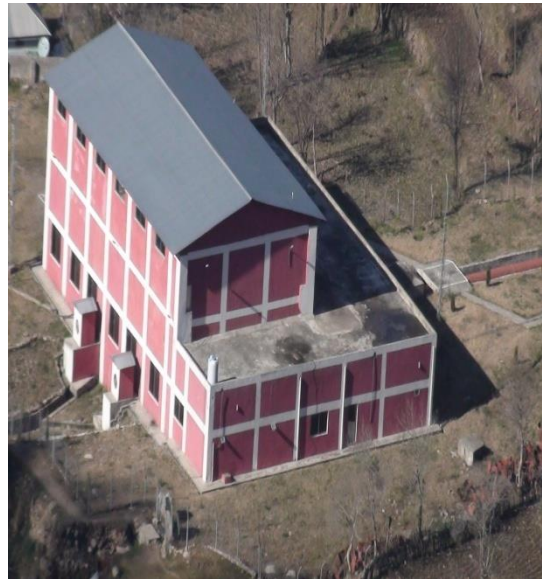
Power House Main building
